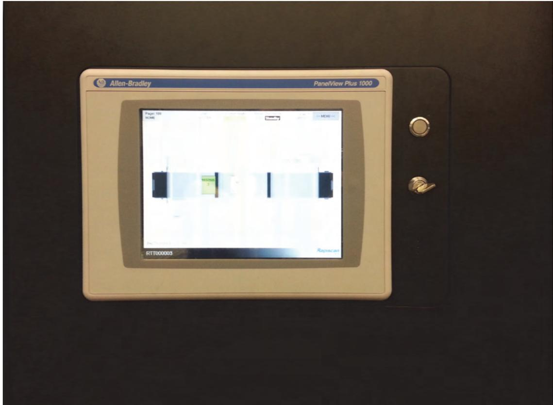
*Figure 2 HMI, Key Switch & Start button*
