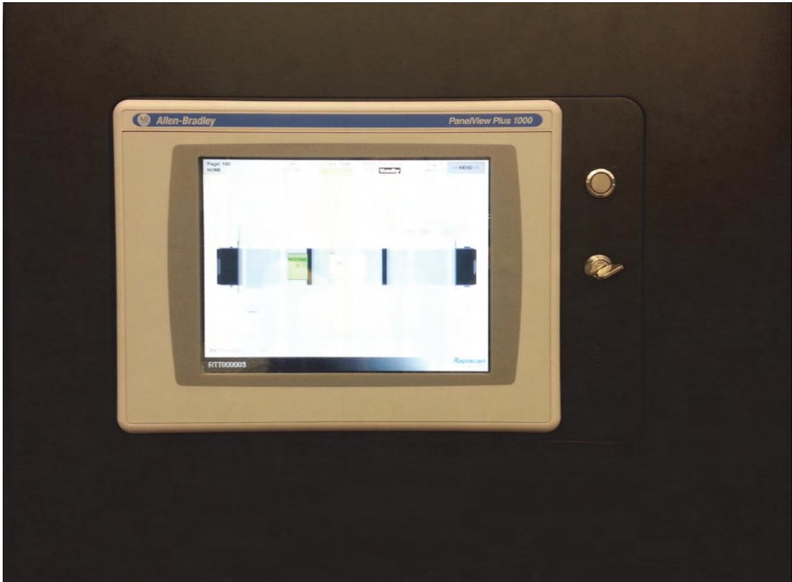
*Figure 8 HMI, Key switch & start button*
