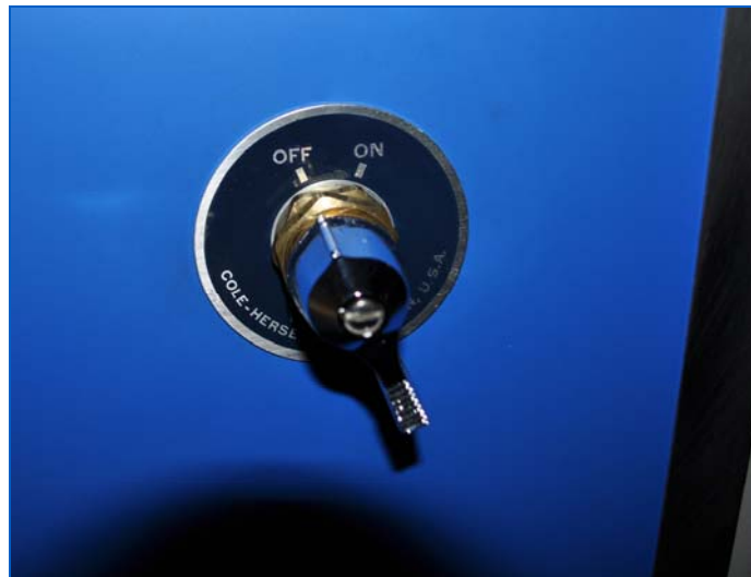
Figure 71: Master Battery Disconnect
