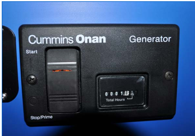
Figure 37: Remote Generator Start Switch
