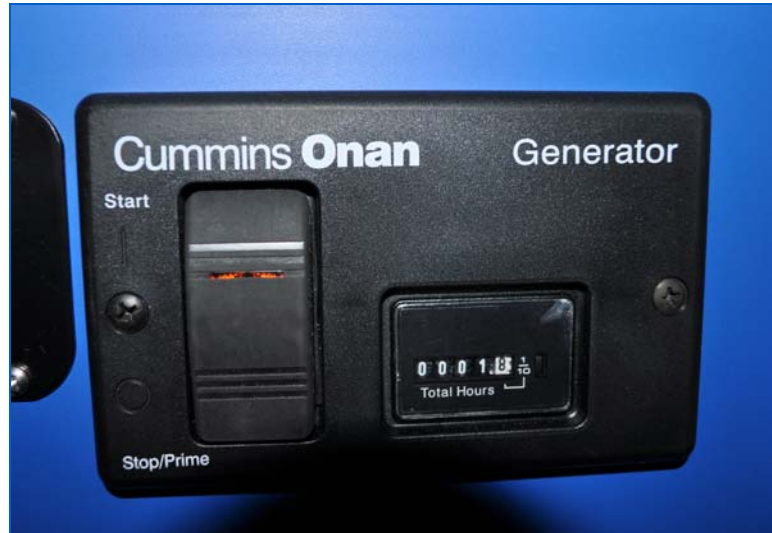
Figure 70: Remote Generator Start Switch
