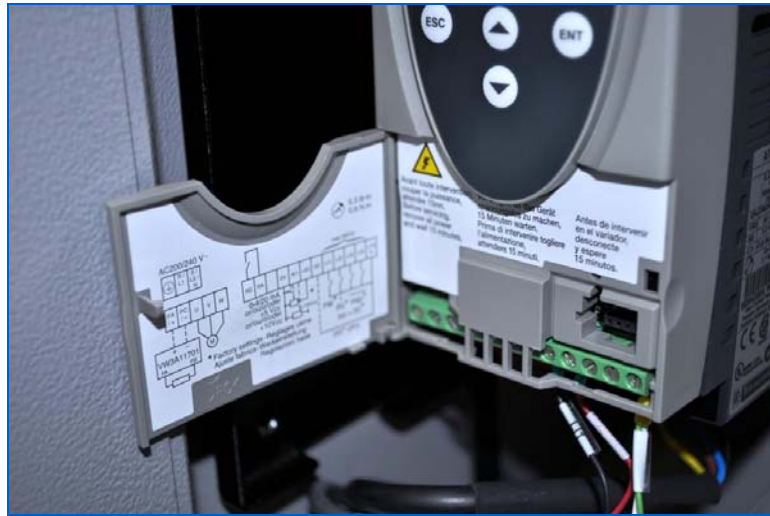
Figure 341: Inverter Terminals
