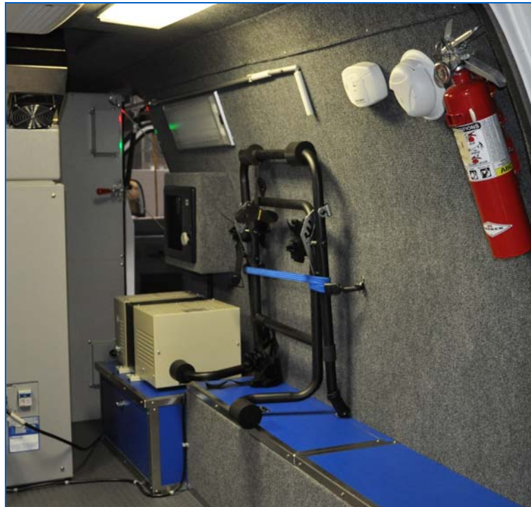
Figure 51: Operator Station Support Rack
