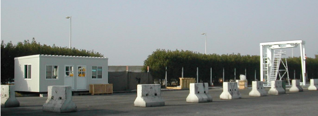
Figure 6. GaRDS Portal Facility
