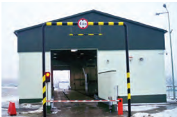
Eagle® G45 within a weatherproof scan hall.
