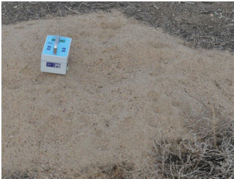
TSA PRM470 hand-held monitor testing construction fill
